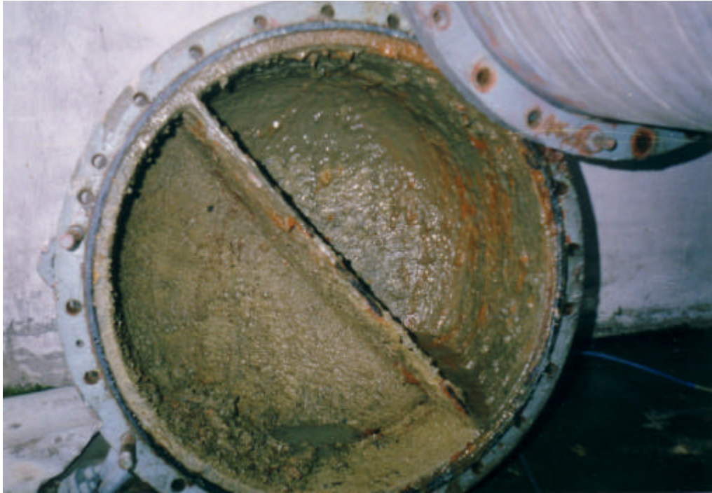
Fig. 10. Ammonia carbamate solution cooler: water turning end prior to washing
