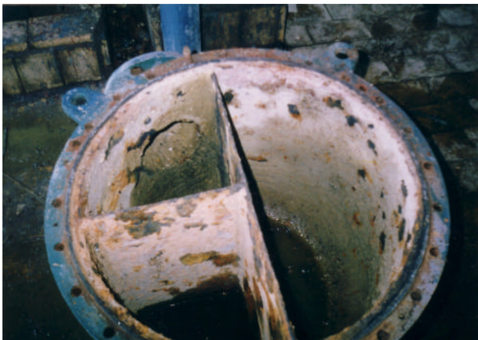
Fig. 12. Ammonia carbamate solution cooler: water inlet head box after washing
