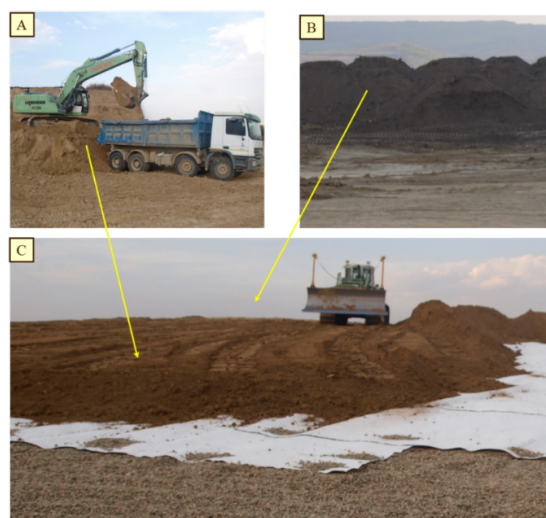
Figure 2. Source of lithogenic and humic soil material for Linic Spolic Technosols under construction
