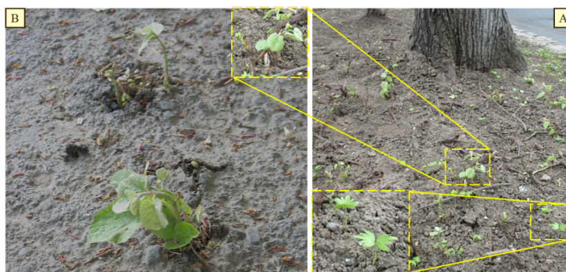
Figure 3. Degradation of asphalt path by deformation cracks and perforation under influence of rooting system of Tillia tomentosa
