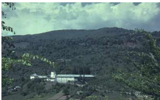
"Stejarul" Research Station in Pangarati (Neamt County, Romania)
